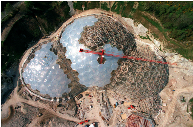
Fig. 17 Erection of the HTBiomes
