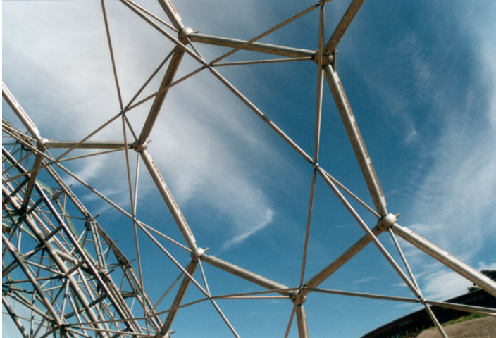
Fig. 4 The Hex-Tri-Hex Structure
