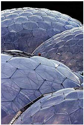
Photo courtesy <u>Apex Photo Agency</u>, Photographer Simon Burt **The giant dome structure of Eden's greenhouse roof dwarfs a** worker installing the transparent panels.
