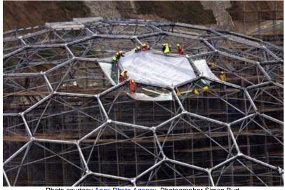
Photo courtesy <u>Apex Photo Agency</u>, Photographer Simon Burt Each ETFE pillow is secured in the steel framework.
