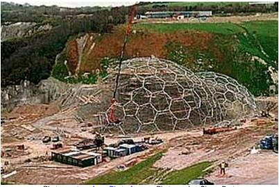
Photo courtesy <u>Apex Photo Agency</u>, Photographer Simon Burt Workers assemble the steel framework of the greenhouses. The Eden Project crew broke the world record for largest freestanding scaffold.
