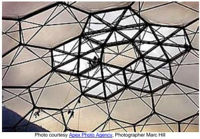
Workers installing ETFE foil panels in the dome ceiling
