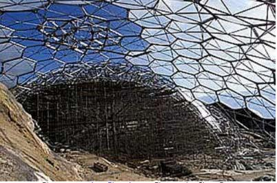
Photo courtesy <u>Apex Photo Agency</u>, Photographer Simon Burt The domes were built along the north side of the pit, so they would get maximum sunlight from the south.
