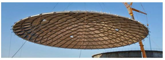
The HMT Geodesic Dome features a clear-span, all-aluminum, lightweight, corrosion-resistant structure which sets a new standard for performance in aluminum geodesic domes.
