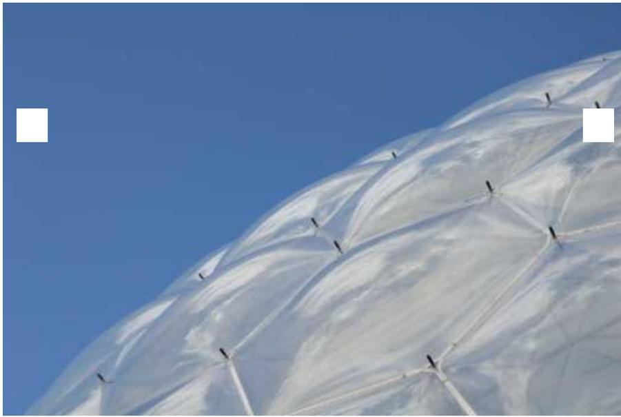
Each hexagonal window has three layers of ETFE.
