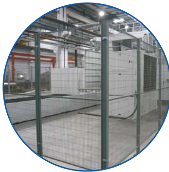
Welded wire fence in a workshop used to protect machines.
