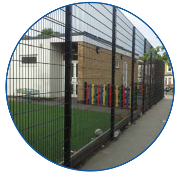
Dense wished welded wire fence is anti-climbing.
