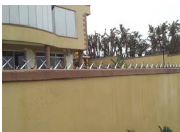
Medium wall spikes building wall.
