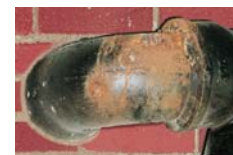
Prevention of corrosion and odour build-up
