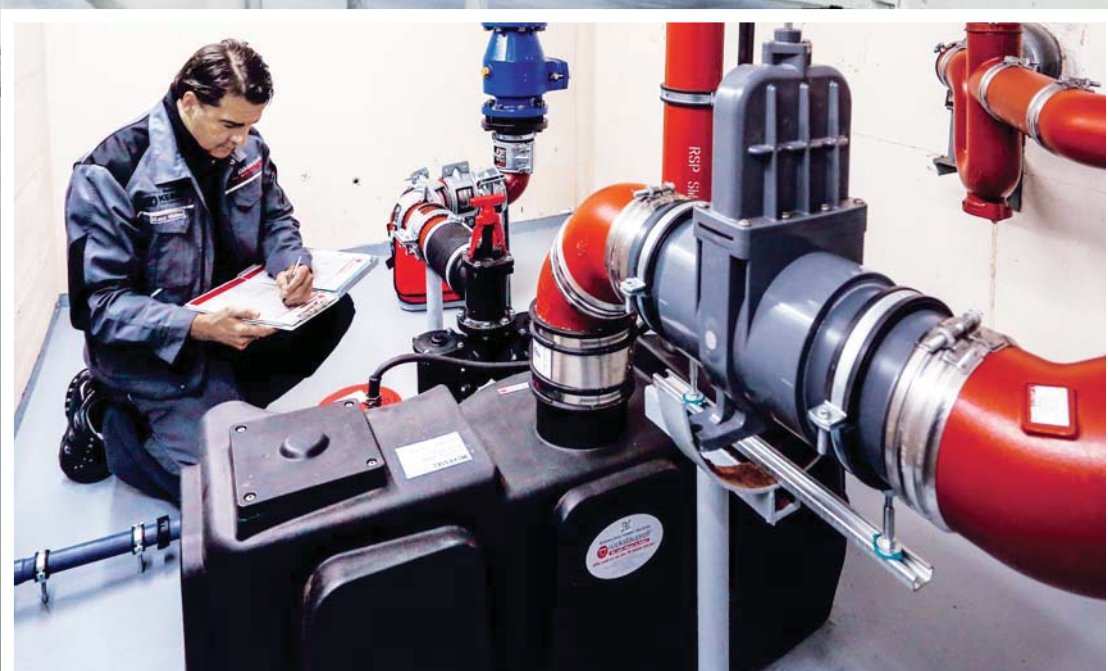
KESSEL-Lifting station Aqualift XL for free standing installation
