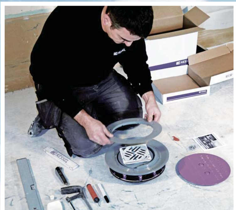
Installation situation Ecoguss project drain with shallow bed waterproofing layer and fire protection
